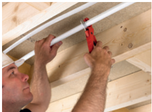
Measure and cut in-situ
