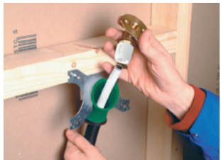
Figure 50: Installation of HX102 terminal fitting plate and HX101/15, 15mm conduit terminal
