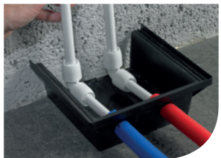
Figure 40: Cut conduit box for wall termination
