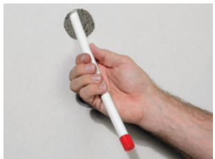
Figure 22: Always protect pipe ends
