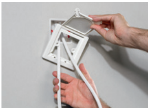
Figure 53: Installation procedure of HX113 cover plate
