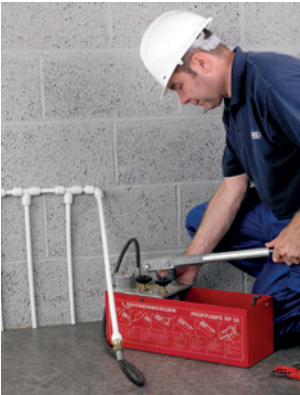
Figure 60: Pressure testing
